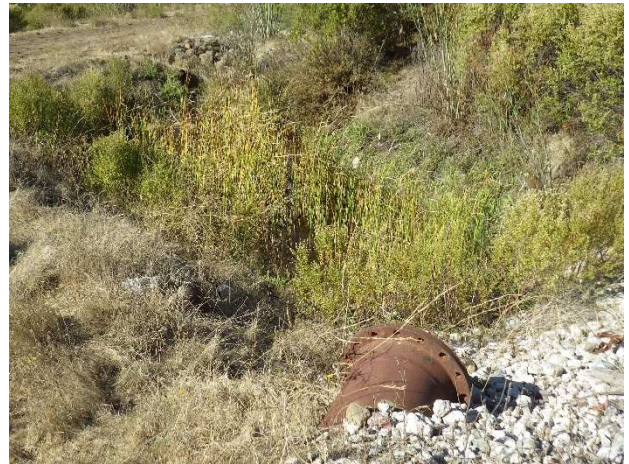
d. Representative photo of Basin 6, taken on April 17, 2018.
